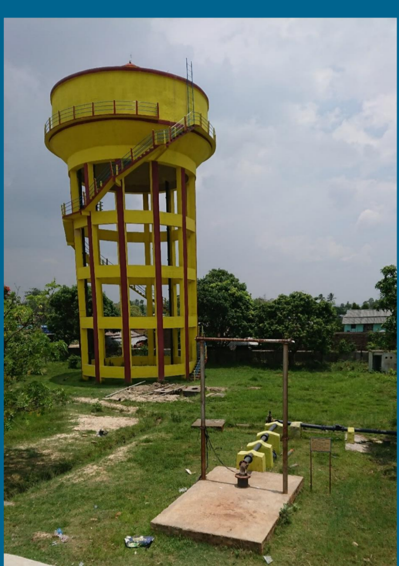
Figure 1: Water tower in Lahan, Nepal
